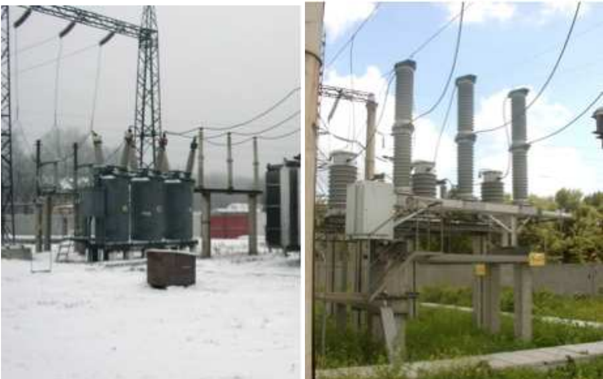
Figure 3. The Circuit Breakers before and after the Reconstruction.
