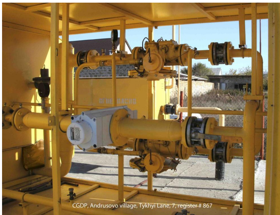
Pic. 2. Repaired CGDP, Andrusovo village, Tykhyi Lane, 7, register # 867
