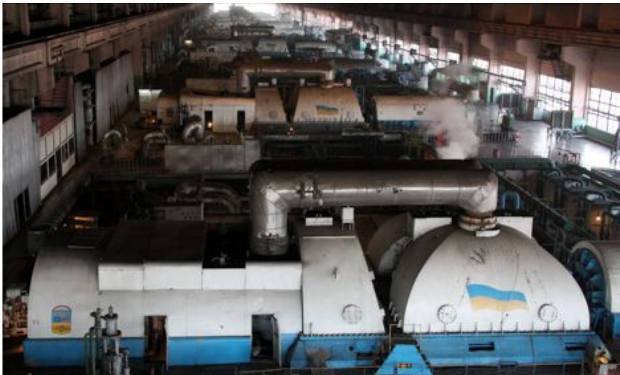
Figure 1. The Turbine Hall of the Kryvorizka TPP.
