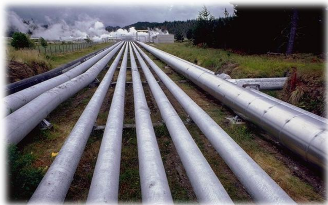
Fig.1. Network rehabilitation with pre-insulated pipes
