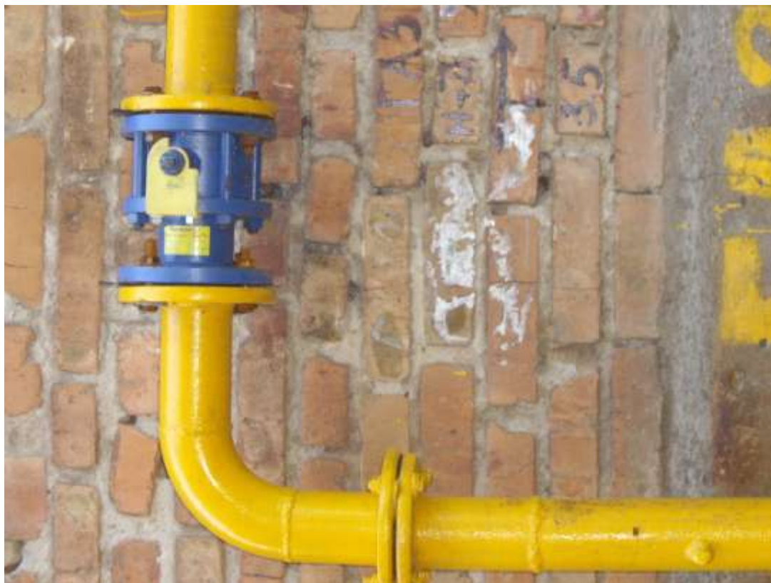
Figure 1. Repaired valve, Kriviy Rih city
