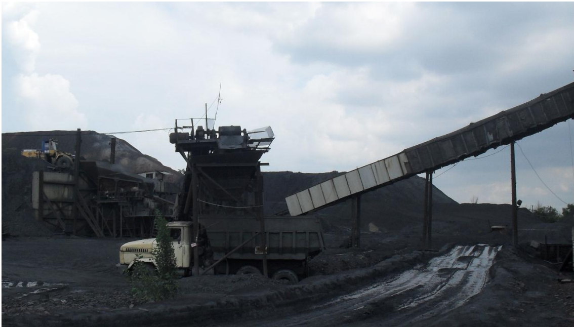
Fig.2 Project activity equipment
