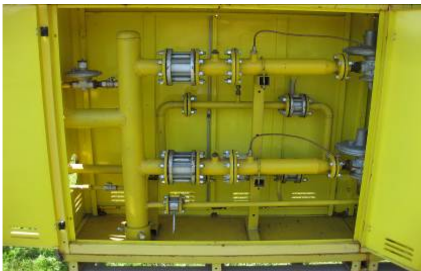
Figure 1. A repaired CGDP, Lubny
