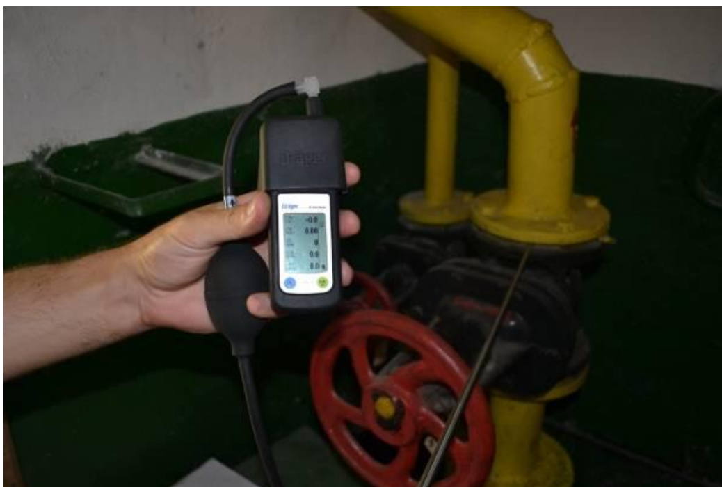
Figure 2. A photo of repairs being conducted, Chernihiv
