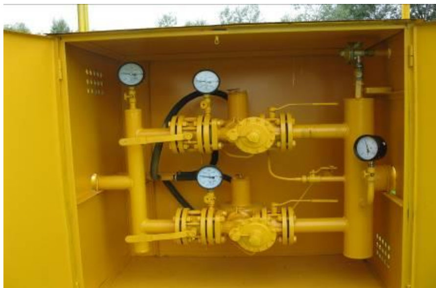
Figure 1. A repaired CGDP, Chernihiv
