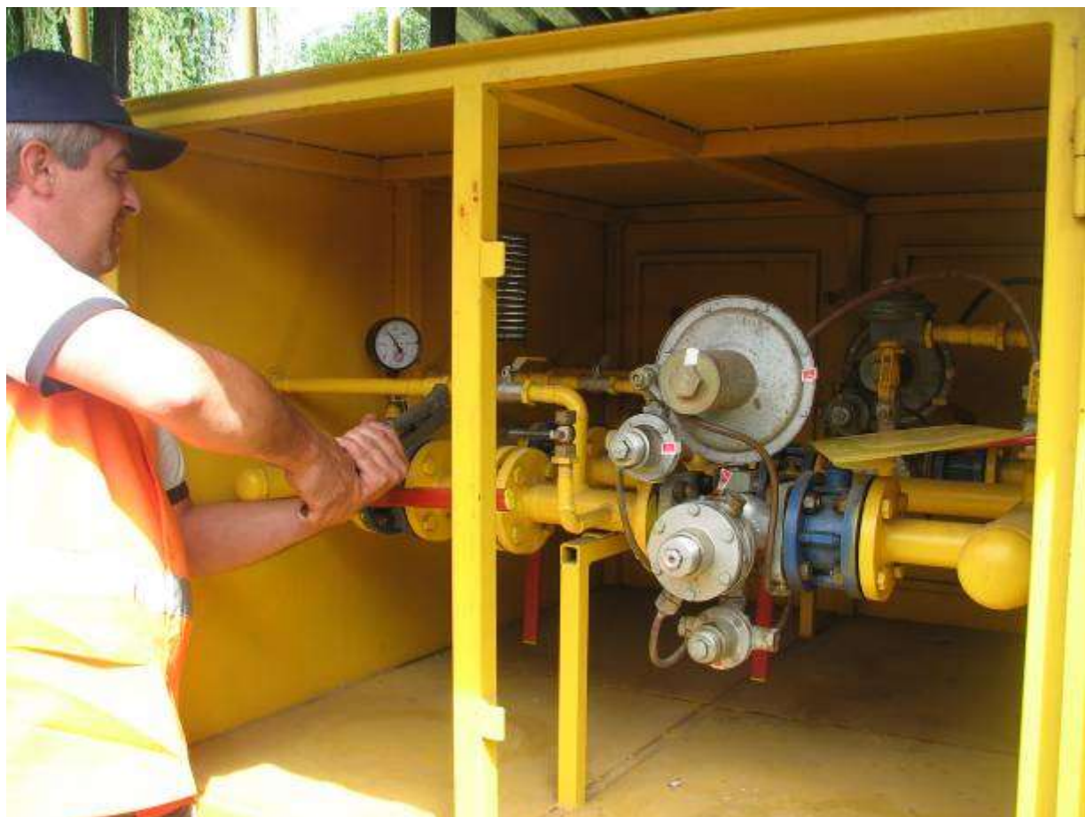
Figure 1. Repaired CGPD, Lubny.
