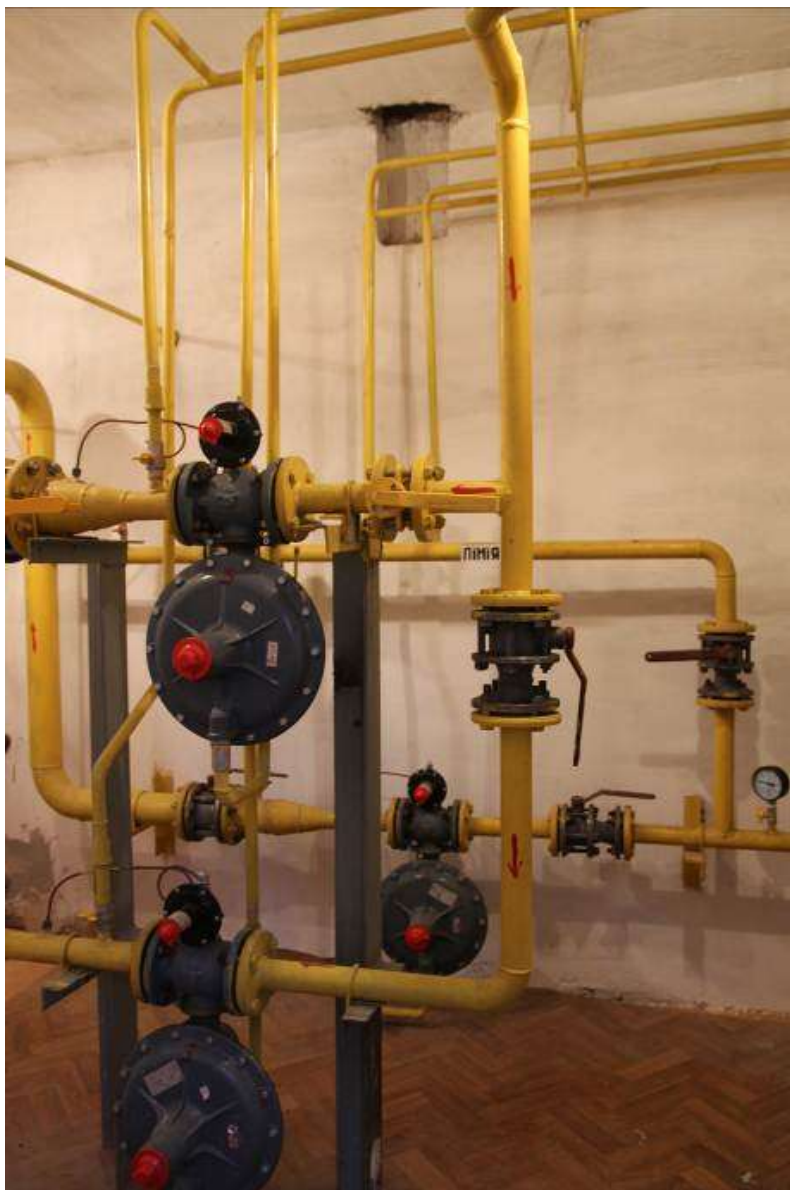
Figure 1. A repaired GDP in Poltava, 28 Gozhulianska St., registry No.458
