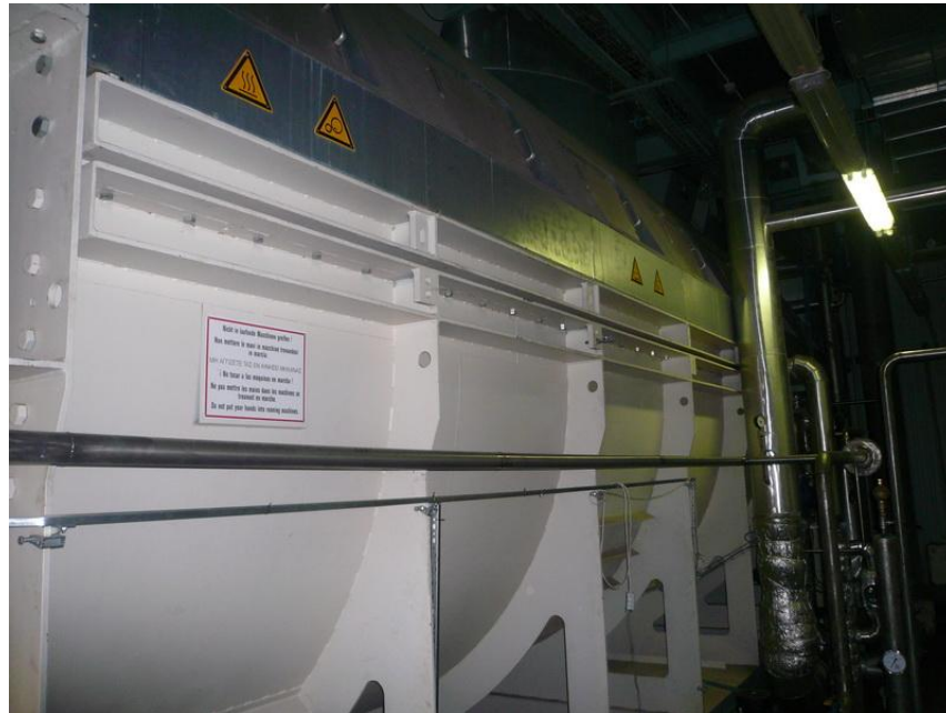
Picture 1.1 The building of drier of beer wort
