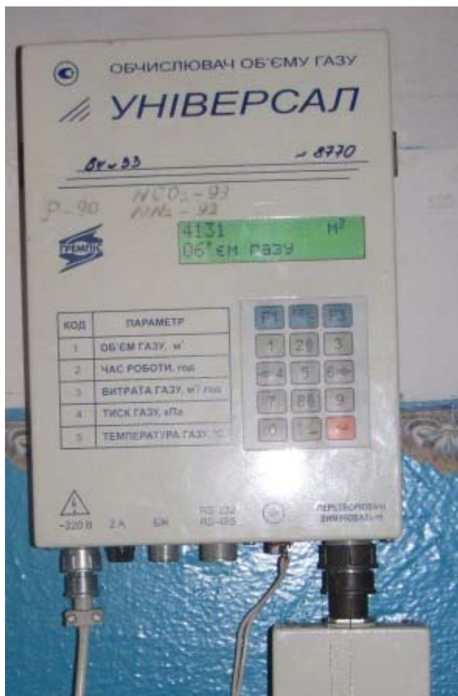
Fig. 1. Installation of gas flow meter with corrector at boiler-house
