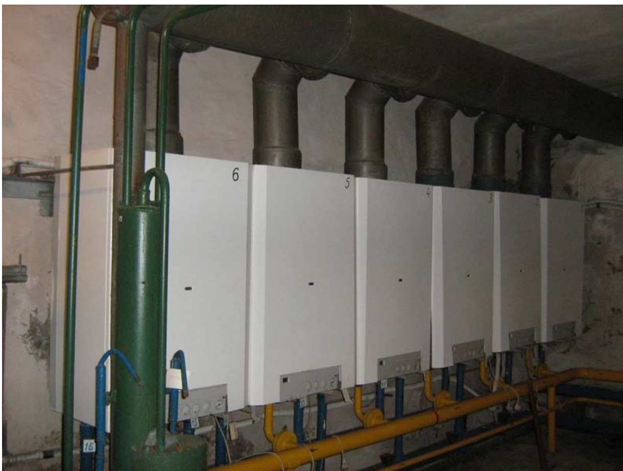
Fig. 1. Reconstruction of boiler-house with modular boilers
