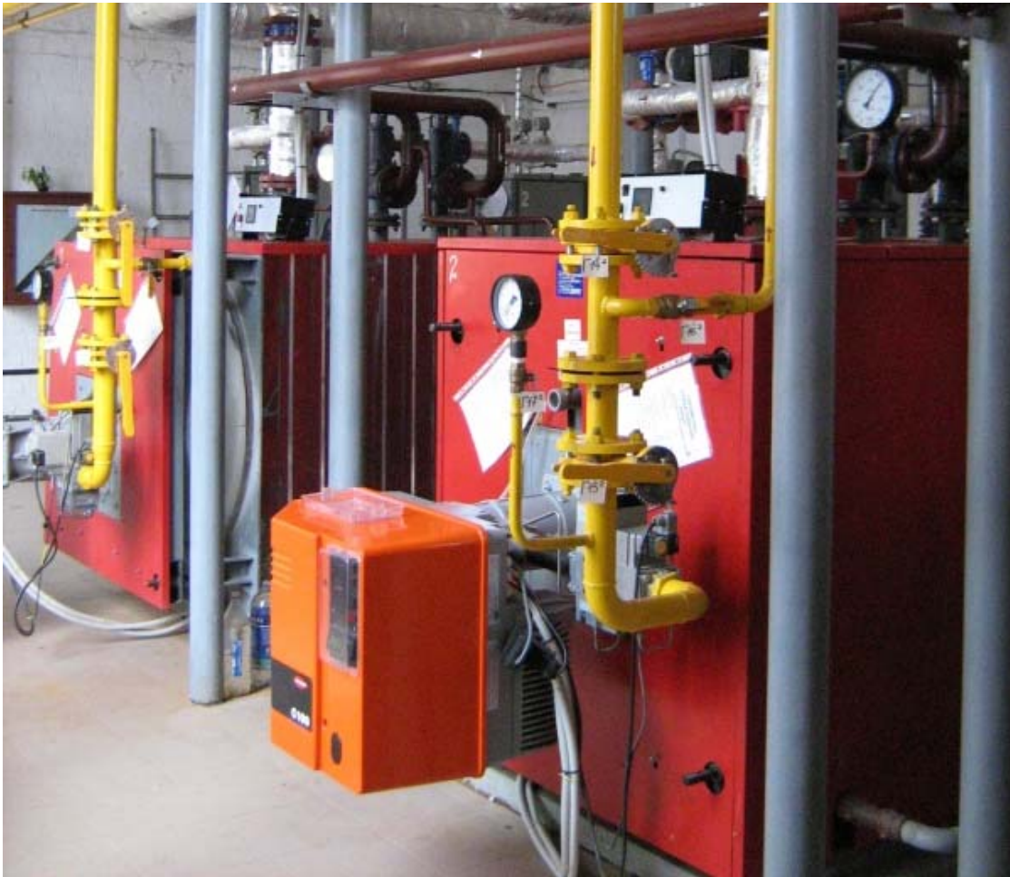
Fig. 1. Reconstruction of boiler-house City Hospital # 6 (#519 in the project) with Kolvi boilers
