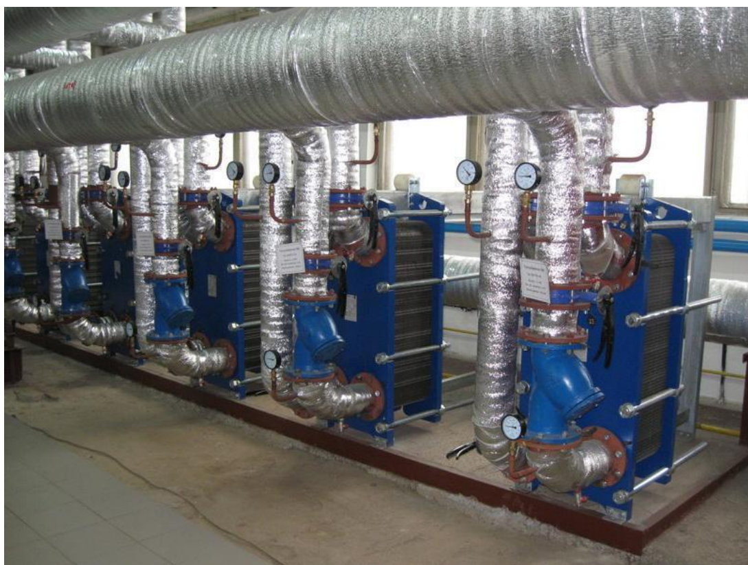
Fig.1. New lamellate heat exchanger
