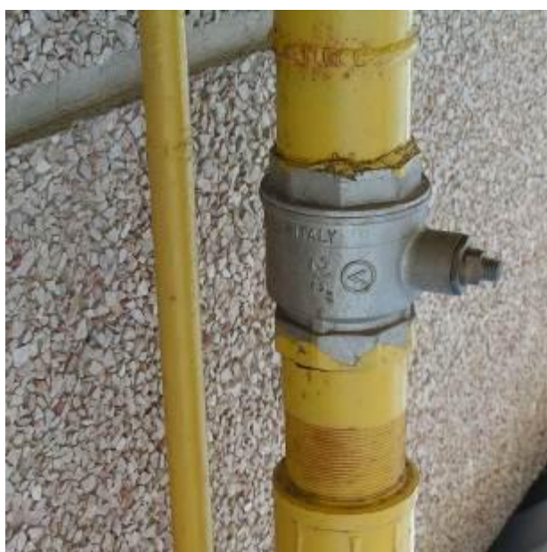
Pic. 1. Gland valve threaded of Italian production
