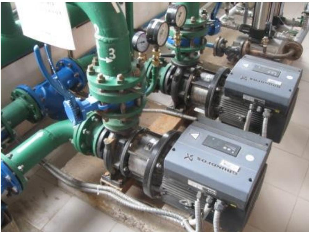
*Fig.1. Step-up pumping station Grundfos CRE1-15 G-A-A-E-HQQE installed at boiler-house Artema, 449b (#102 in the Project)*
