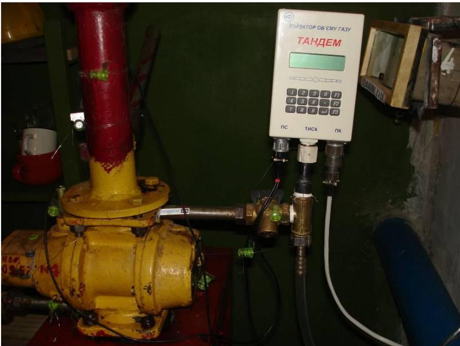
*Fig. 4. Gas flow meter with corrector*
