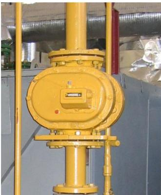
*Fig. 3. Gas flow meter*
