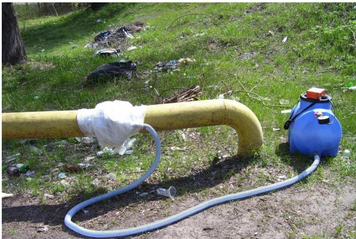
Picture. 1. Photo of a plant for quantitative measurement of methane leakage.
