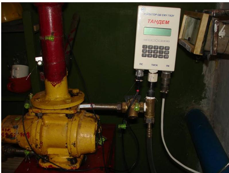
*Fig. 3. Gas flow meter with corrector*
