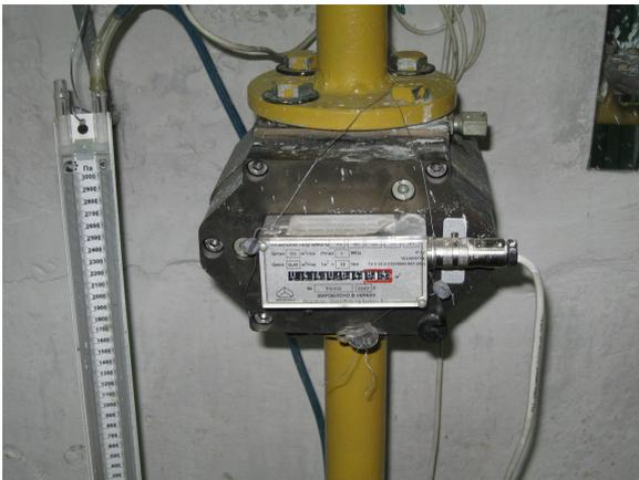
*Fig. 2. Gas flow meter*
