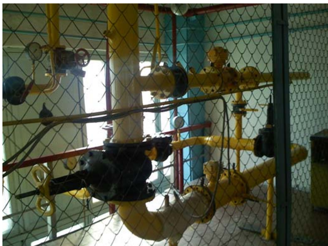
Fig. 1. Gas distribution unit
